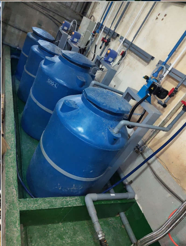
Waste Water Treatment System at Art Furniture Co., Ltd - Flow rate 72m 3 /day
