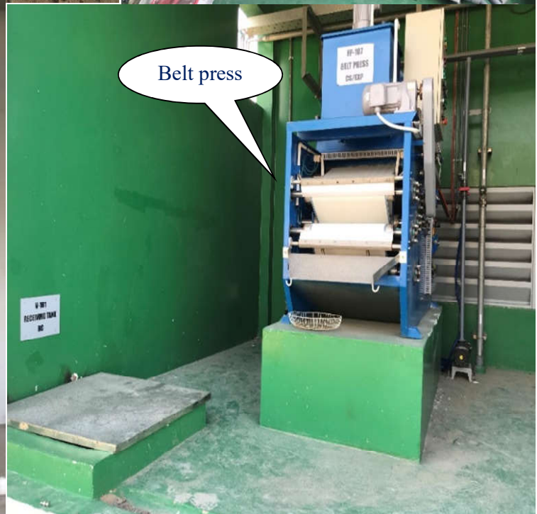
Sewage water treatment system at Great Kingdom Giang Dien – Factory A 150m 3 /day
