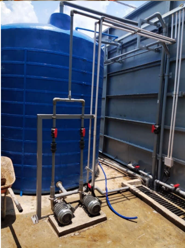
Waste Water Treatment System at Art Furniture Co., Ltd - Flow rate 72m 3 /day
