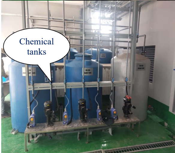
Wastewater treatment system at Great Kingdom Giang Dien Factory B - Flow rate 284m 3 /day.
